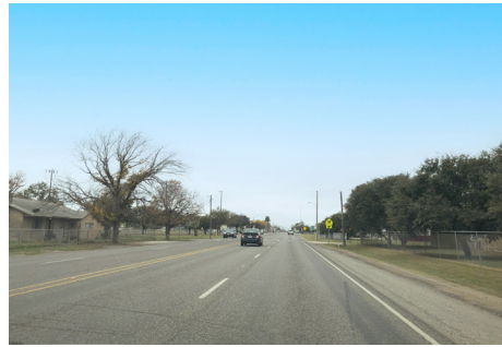
Image 1.5 - Four-lane US 57 Section in La Pryor
