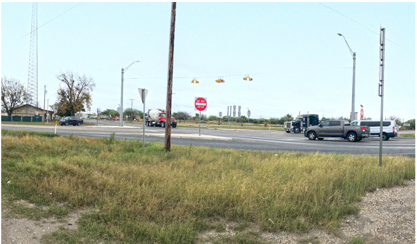
Image 1.8 - US 57 at US 83 Junction in La Pryor (Looking Southeast)
