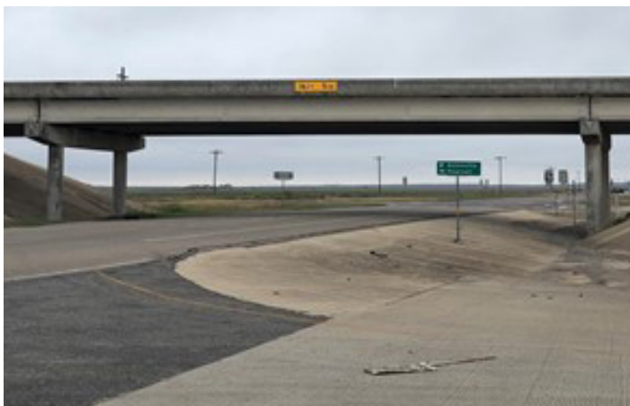
Image 6.1 - US 57 at FM 140 Bridge Clearance
