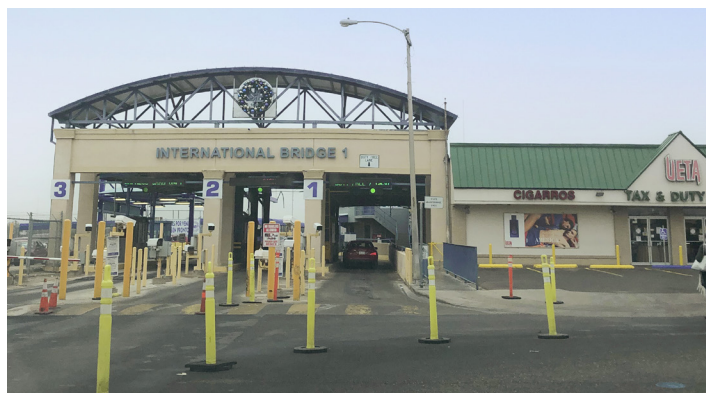
Image 1.2 - Bridge I in Eagle Pass
